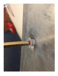
**NOTE:** The time of year you are fitting can impact on the tightening step of the process. If it is cold, then tightening to the 2-3mm recommended is pretty straight forward.
