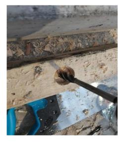
Put in 16mm Augur/Wood bit and drill through to the ground.
