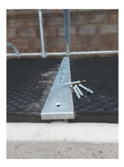
Using a 10mm drill bit, drill a hole into the concrete (go a minimum of 80mm into the concrete) using the strip as the template and push a frame fixing in it's sleeve into the hole before proceeding to drill the next one. Do not separate the screw from the sleeve. Marking the drill bit at 110mm will let you know when it is far enough down as you won't be able to see 80mm due to the strip.
