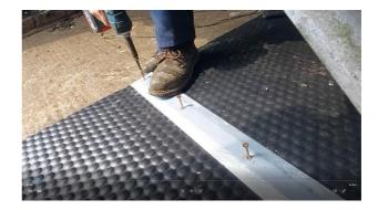
Make sure that the sleeve of the frame fixing is in contact with the strip and the head of the screw as this helps to prevent corrosion
