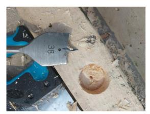
Mark the timber where you are going to put a fixing. Using your 38mm wood bit, drill a hole in the centre of the brisket board to a depth of 1" (to countersink the head of the fixing)
